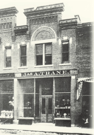
Trane Storefront La Crosse, Wisconsin 1891
